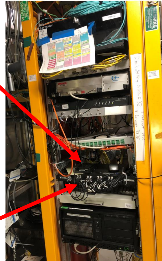
LEMO cables from high-n array mag probes
